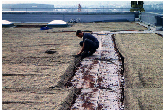
Figure 5 Laying of jute netting over green roof areas that are prone to wind erosion.
