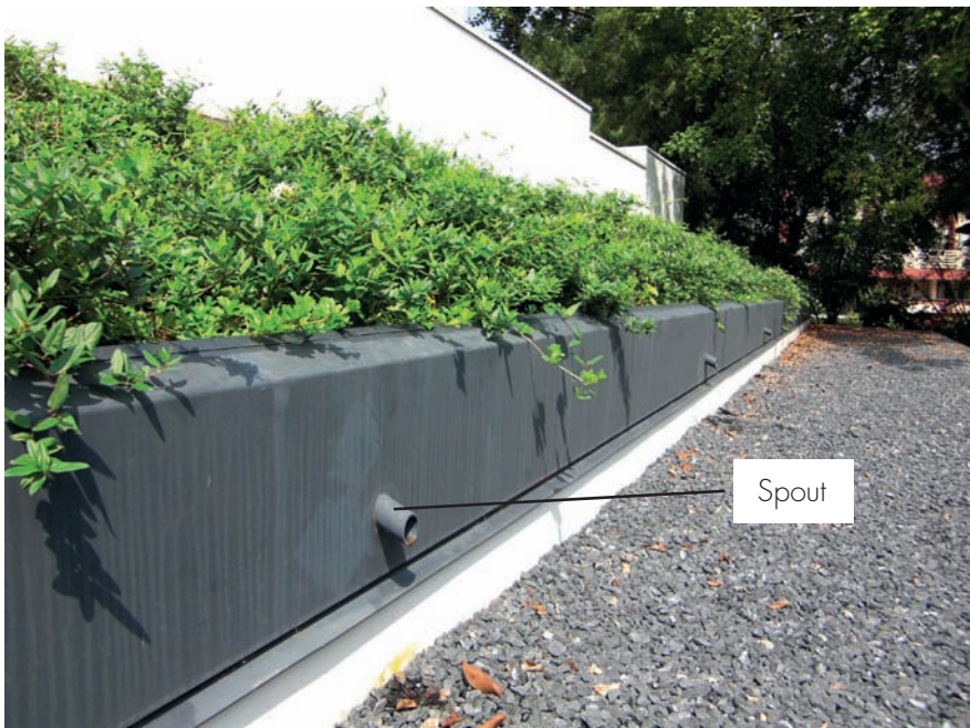
Fig 16: Spouts along the shear barrier of the pitched green roof.
