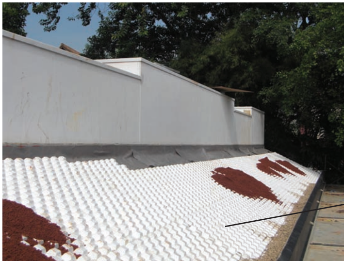
Fig 6: "Protruding teeth-like" intermittent shear barriers as integral parts of the pitched green roof system.
