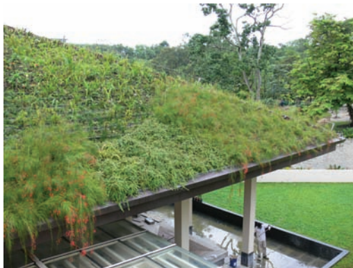
Fig 13: Singapore Botanic Gardens, Singapore. The vegetation is a mixture of shrubs and ground-covers, irrigated by an automatic system. This pitched green roof is only accessed during periodic maintenance. There are safety life-lines along all four hips of this roof.
