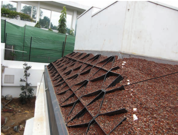
Fig 10: Plastic substrate-retainer rigid structure that is appropriate for steep slopes of 20^{\circ} to 45^{\circ} .
