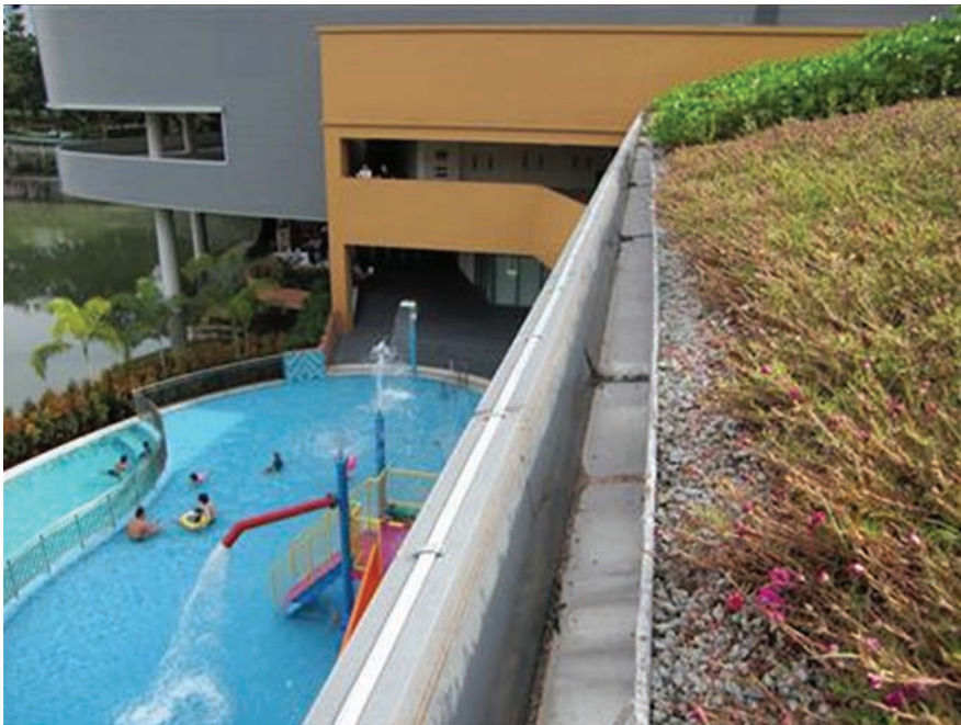
Fig 15: Open gutter at the sloping green roof at Cashew-Senja Community Club.
