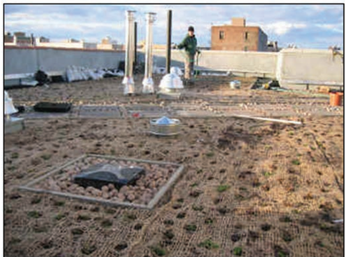
Fig 4: A green roof that is over laid with jute netting.
